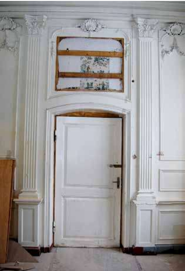
(1) In situ research. The uppermost layer can be separated from the lower ones by a prophylactic layer made of Japanese paper. Photo by Andreja Dragojevic (2) Older wallpaper layers can also be displayed as sample areas. Photos by Kadri Kallaste (3) Wallpapers surviving in their entirety can often be found behind panelling. The neo-Rococo panelling in the dressing room of the countess of the Puurmani manor revealed a beautiful Chinoiserie wallpaper (4) A wholly surviving 1930s wall scheme discovered during interior finishing work at Roopa 11 in Tallinn
