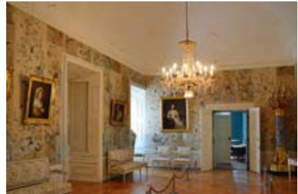
Figure 148. Final outcome after remounting the restored wallpaper panels.
