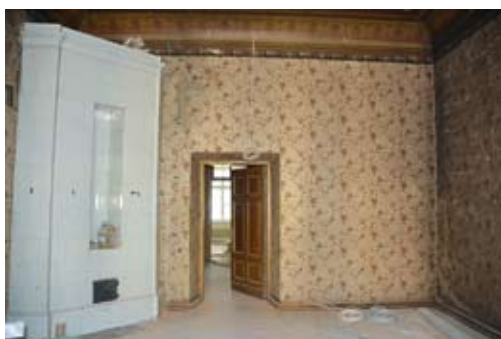
Figure 184. Papered room before restoration.
