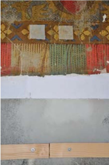
Figure 127. Patches of Japanese tissue to add additional protection.
