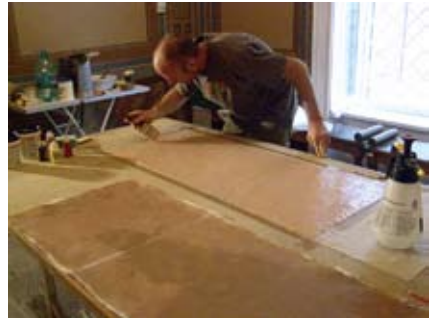
Figure 137. To reproduce the embossed effect of the wallpaper, a silicone mould needed to be taken.
