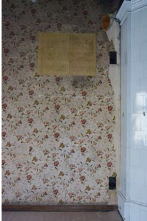
Figure 155. Large segment of wallpaper removed from the wall prior to restoration.
