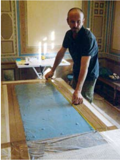
Figure 137. To reproduce the embossed effect of the wallpaper, a silicone mould needed to be taken.
