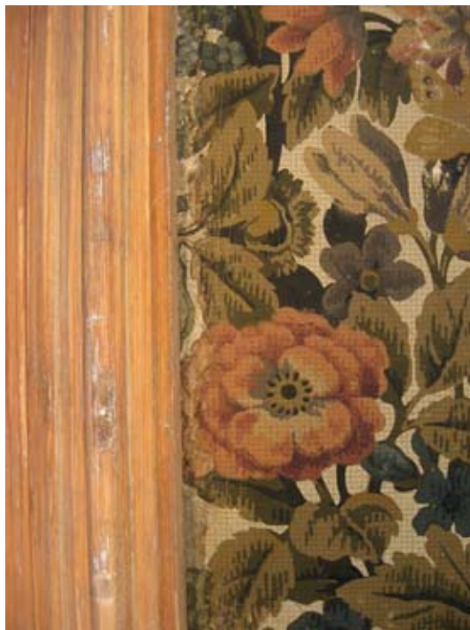
Figure 101. Missing areas in the wallpaper of the Puurmani manor's dining-room were integrated into the rest with the help of modelling lines in matching tones.
