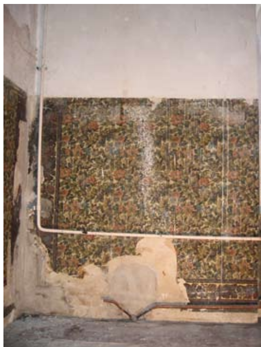
Figure 170. Condition of the wallpaper after the removal of the wooden paneling.
