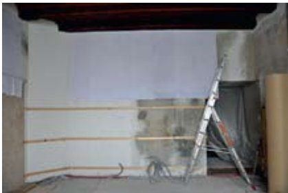
Figure 126. Walls were covered with a layer of acid-free lining paper prior to remounting.
