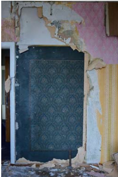
Figure 61. Three part wallscheme found in a wealthy middle-class apartment in Roopa 11, Tallinn.
