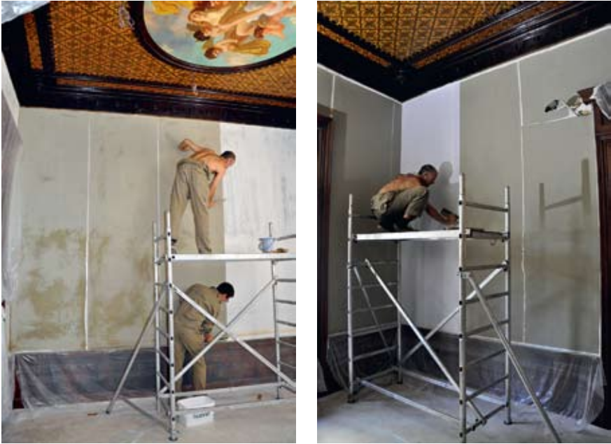
Figure 99. An easily removable mounting system was built up in the Theodor Aman Museum in Bucharest. It consisted of a layer of thin cotton canvas and two layers of non-acid lining-paper.
