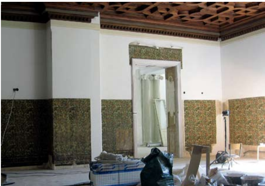
Figure 115. After removal of the wooden over-doors, large fragments of wallpaper and border were discovered.
